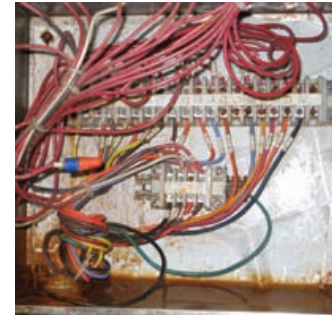
Water accumulation in electrical cabinet
