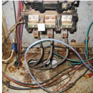
Corrosion leads to premature component failure
